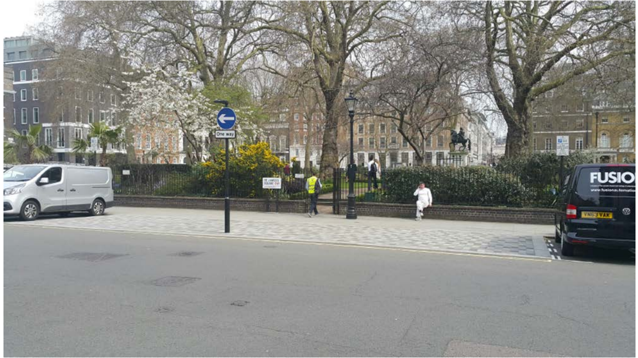
Footway on the south-west side of St James Square, opposite the junction with King Street
